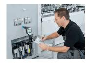
Oil, water or particles in compressed air have a negative effect on the service life of pneumatic components. Energy and operating costs rise, and in worst-case scenarios can lead to unexpected production downtime. Centralised and decentralised measurement of the compressed air quality includes inspecting the service units, measuring the water and oil content, air temperature and pressure as well as determining the pressure dew point.
