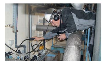
Leakage detection in the plant in Koog aan de Zaan. The detected leaks represent about 8% of total compressed air costs.
